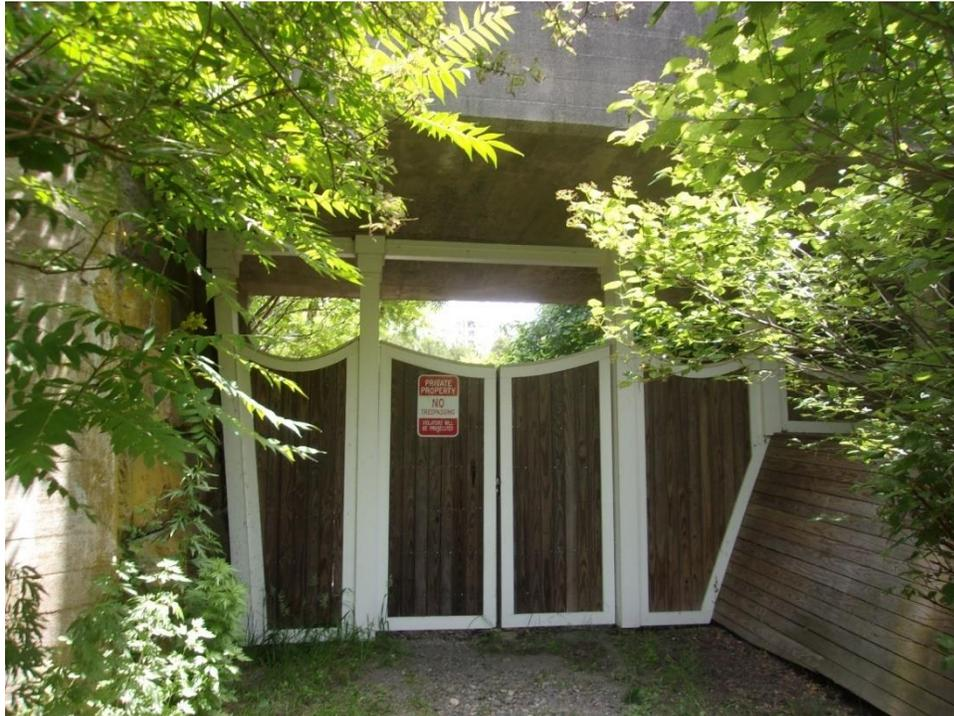
West elevation view of the existing reinforced concrete slab railroad bridge and granite stone abutments. One alternative bikeway option could be constructed on top of this structure. The wooden paneling to the right conceals sewer piping.
