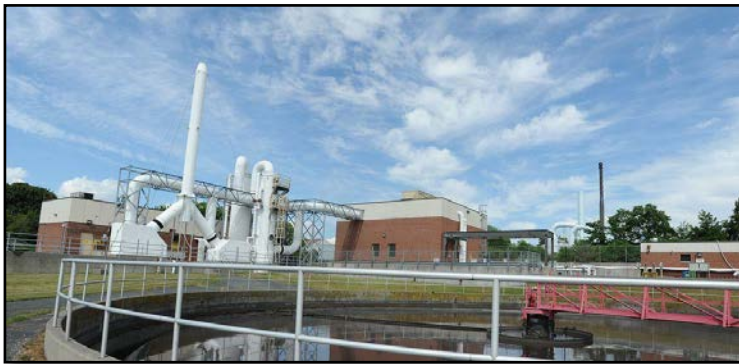
Fall River Wastewater Treatment Plant
