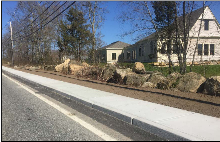
New sidewalk along Bulgarmarsh Road
