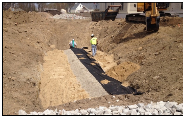
Bio-retention drainage system installation
