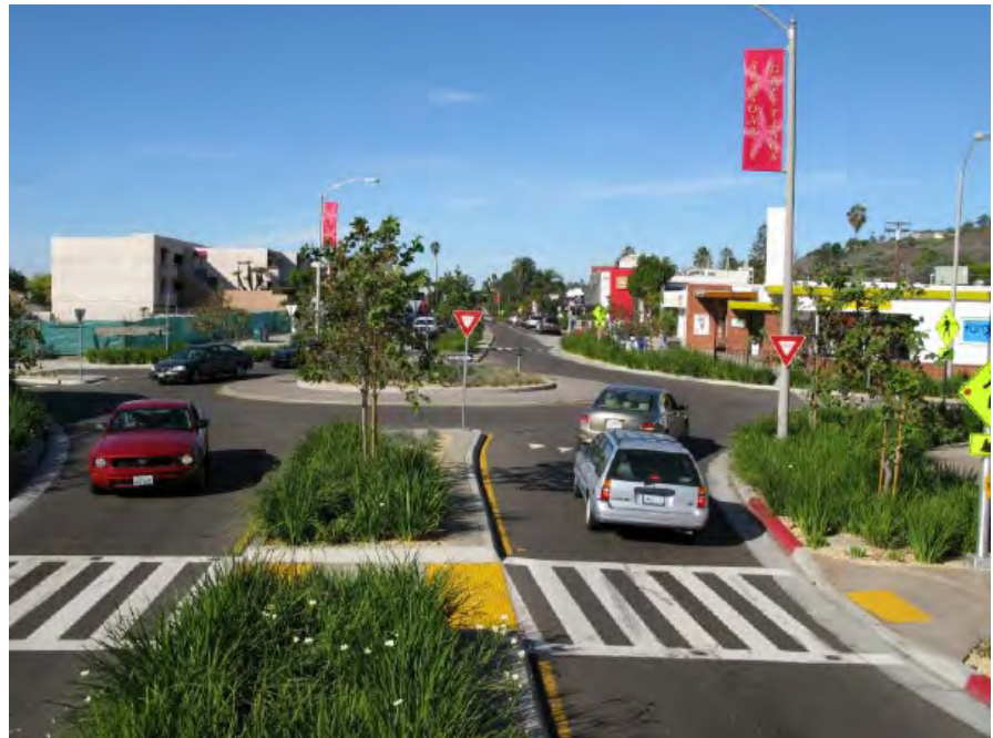
Roundabout: San Diego, CA (Credit: Michael Wallwork)
