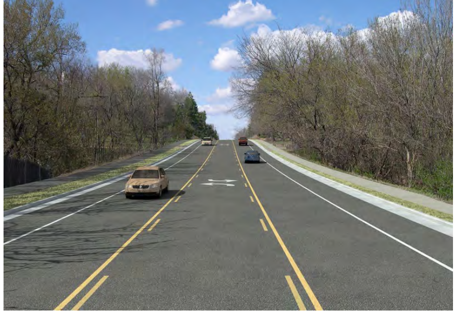
Center-turn lane (Credit: URS)
