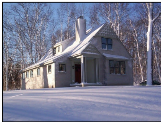
Most homes in Tiverton are single family detached structures
